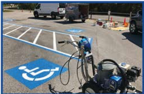
Parking Lot Striping
